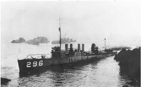
Photo # NH 86411 USS Chauncey and other ships wrecked at Honda Point, Sept. 1923
